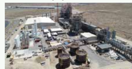
Fulcrum's currently under construction SAF production plant (as of Jun 2020)
