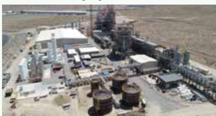
Fulcrum's currently under construction SAF production plant (as of Jun 2020)
